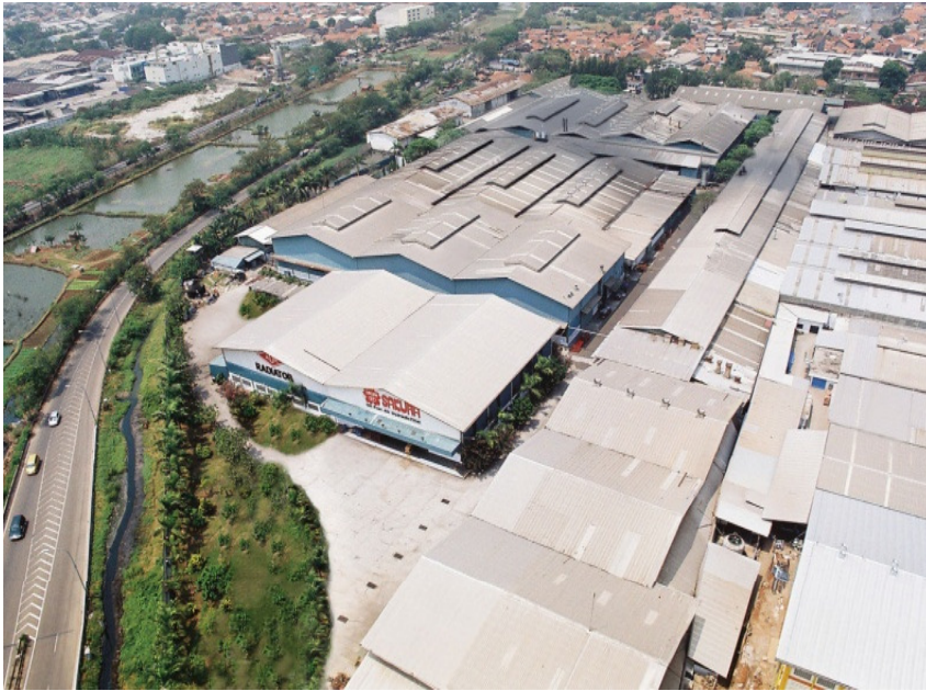
Kapuk Plant (Radiator Facilities)
